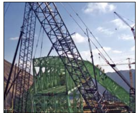
Grove rough-terrain cranes and Manitowoc crawlers are providing construction support.
